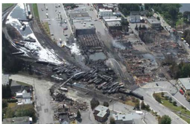
Credit: Transportation Safety Board R13D0054
