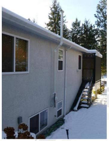
Proven mitigation method Catch radon & dump outside Low wattage fan
