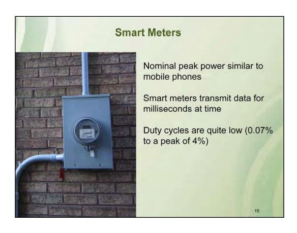
The smart meters transmit data four to six times a day for milliseconds at a time, therefore the duty cycles are quite low (0.07% to a peak of 4%)
