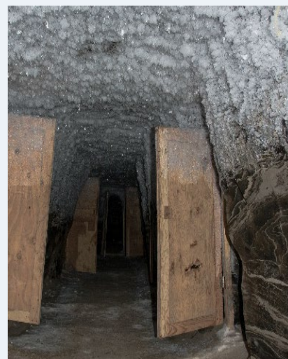
Underground freezers in Tuktoyaktuk
