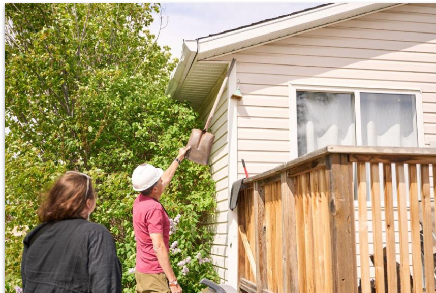
Photo Credit: Indigenous Clean Energy
