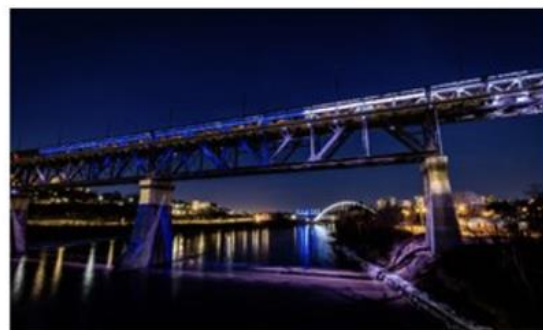
Edmonton High Level bridge, November 25th
