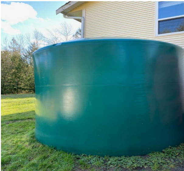
Figure 1: Household 2500-gallon cistern for private well water storage. (Credit: A. Eykelbosh)
