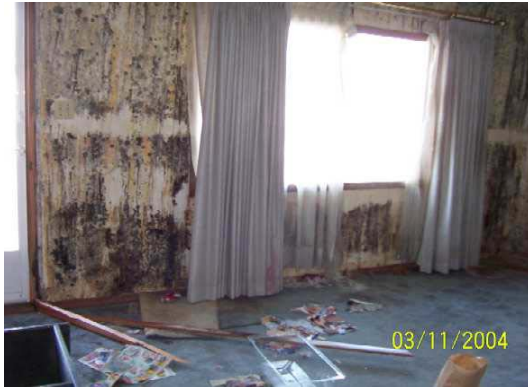
Fig 3-14 Mould – Photo A
