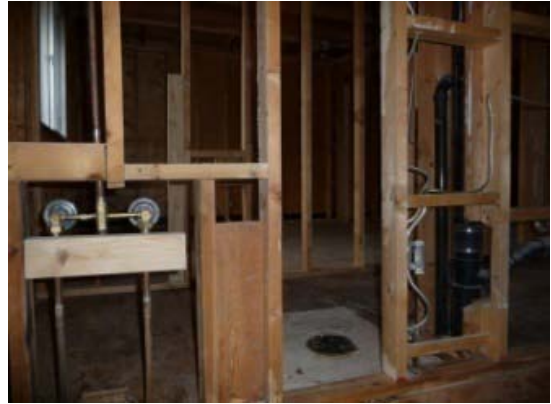
Fig 3-10 Drywall removal
